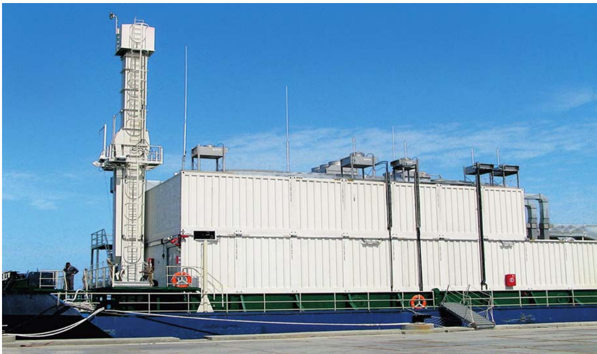
Front-section of an offshore H 2 S-TR shelter, Kazakhstan
